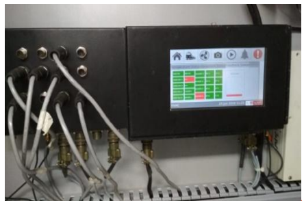
Fig.9: Heating Ventilation & Air Conditioning Unit
